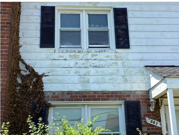
CMU spalls and staining
