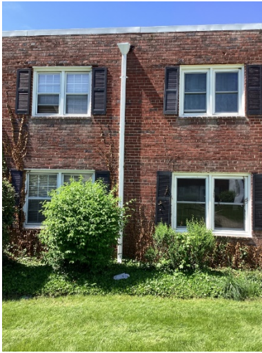
Aluminum downspout and scupper overview
