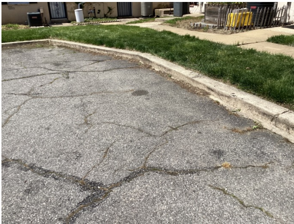
Concrete curb overview
