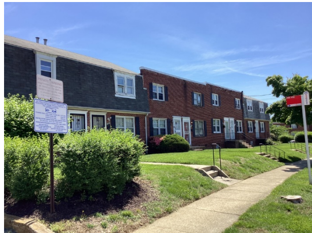
Front elevation overview
