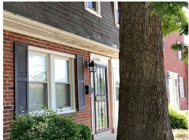
Wall mounted light fixture
