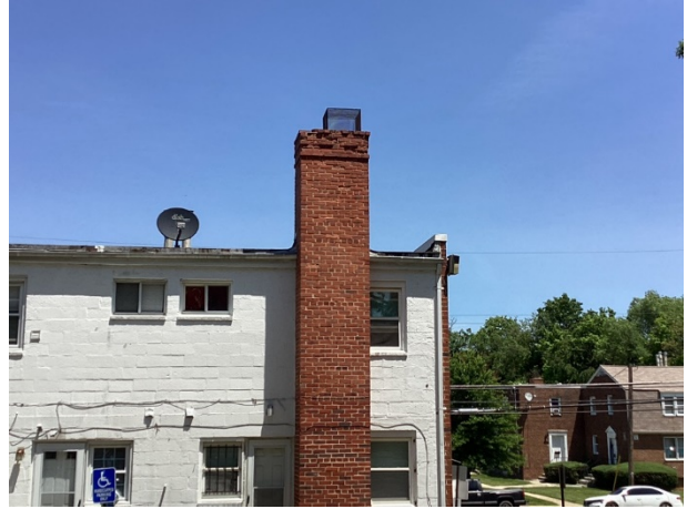
Masonry walls overview
