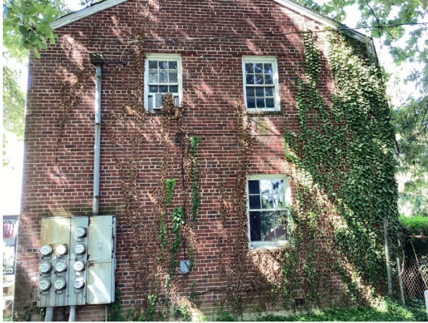
Masonry walls overview
