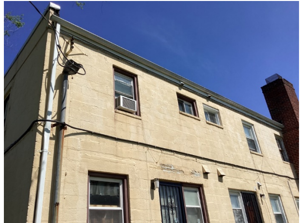
Aluminum gutters and downspouts overview
