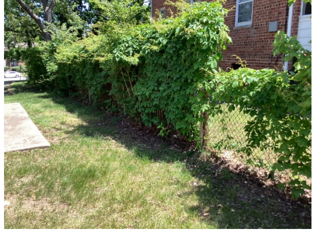
Chain link fence overview
