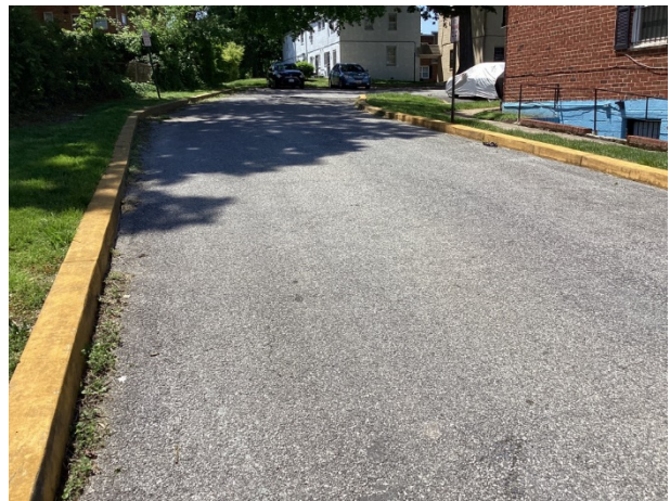
Asphalt pavement parking lot overview
