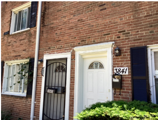
Exterior light fixtures
