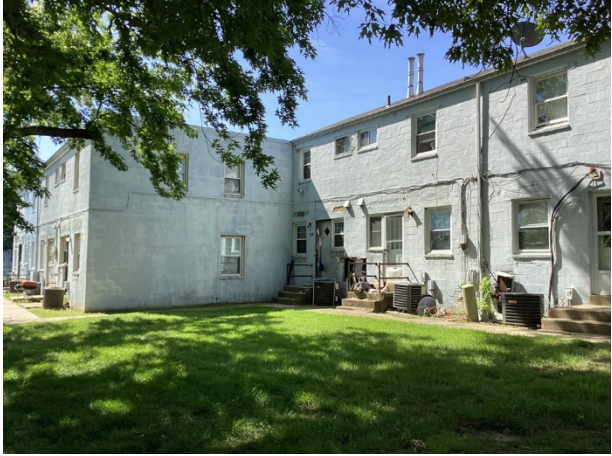
CMU block overview
