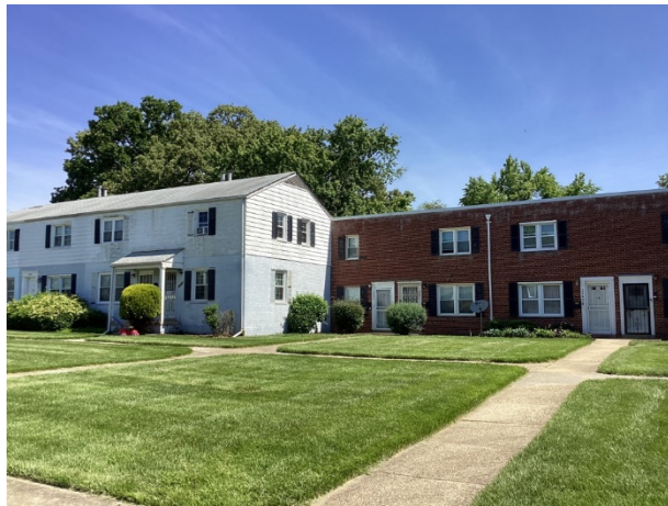
Front and side elevation overview
