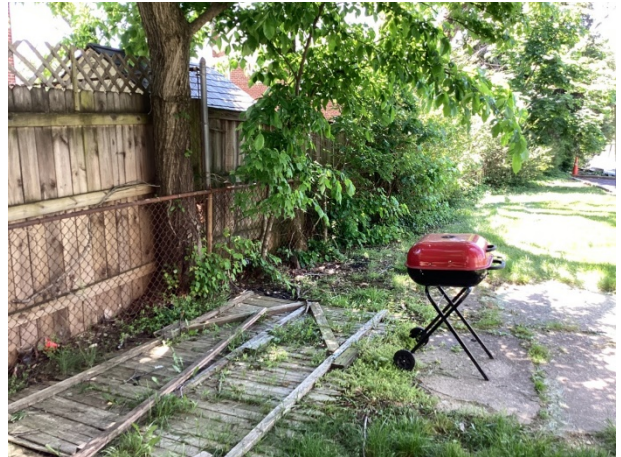
Chain link fence overview
