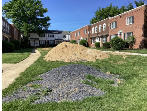
Subsurface utility pipes repair
