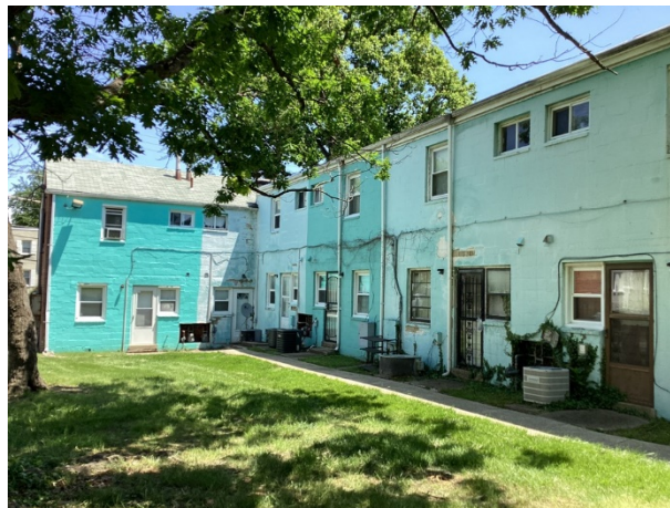
Rear elevation overview
