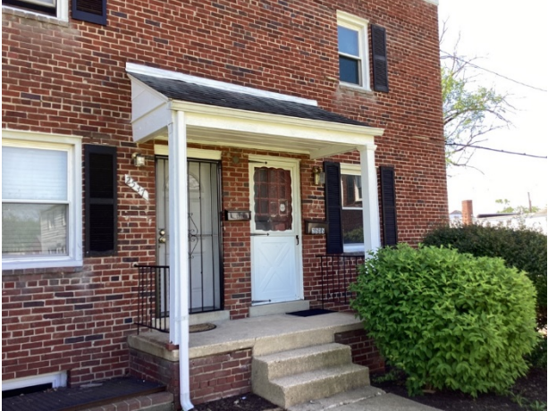
Portico roof overview
