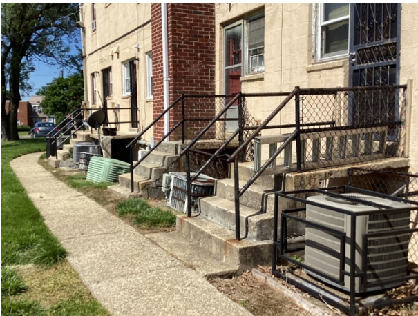
Concrete stoops overview
