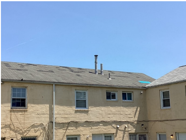
Roof overview with replacements
