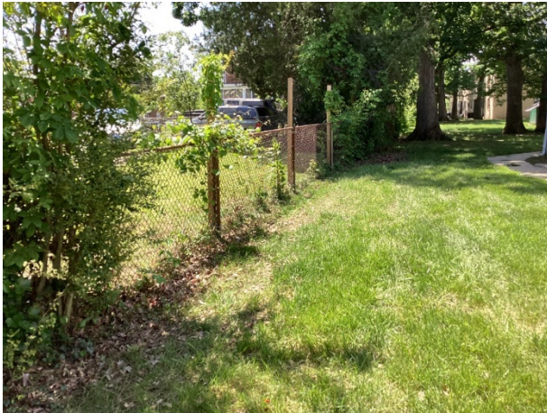
Chain link fence overview
