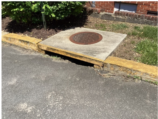
Catch basin overview
